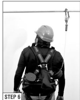
STEP 6 After Lateral Movement Change the SRLs leg for making lateral movement between the anchor points & this can be done with 100% tie-off assurance.
