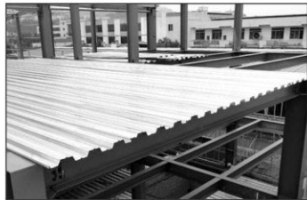
Steel deck and metal roofing
