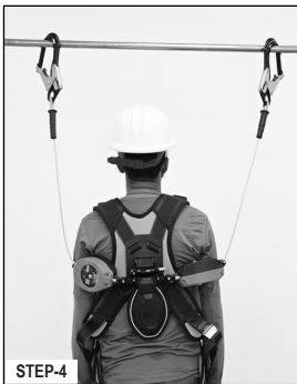
STEP-4 Ensure that both legs are connected to successive anchorage points for lateral movement.
