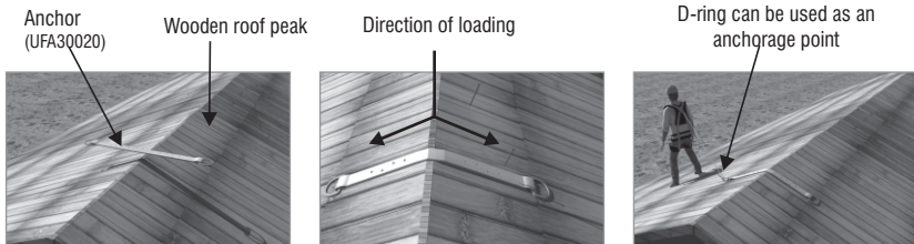
Fig.1- Wooden roof structure on to which anchor is to be installed.
